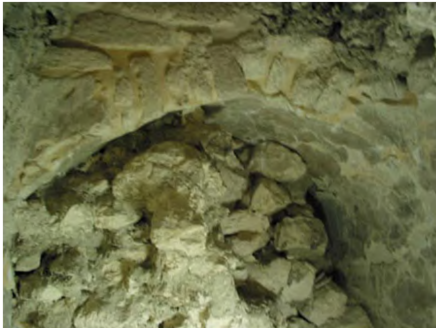
Photo 8. View of circular depressed vault, Sub II c-2, Calakmul.
