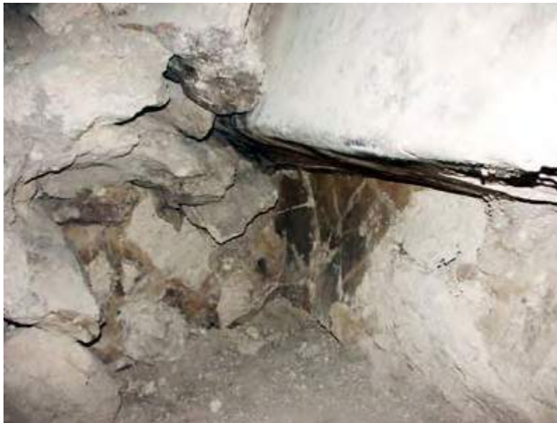
Photo 10. Detail of moldings, bodies of basal platform, Sub II c, Calakmul.
