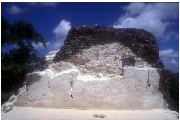
Figure 18. West wall of Room 4 after excavation. Note channels picked through plaster to expose joins in the limestone block masonry.
