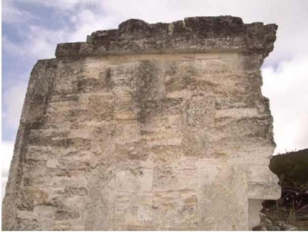
East room, north façade with recessed panel.
