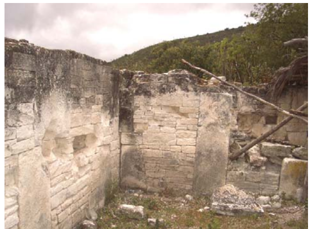
Southeast corner of the patio. The veneer facades were built with blocks of various sizes
