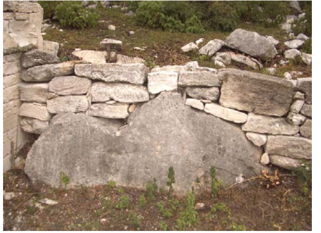
East wall of patio (recent addition).
