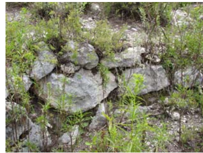
Retaining wall of an artificial terrace in the southern slope of Cerro Coscomate
