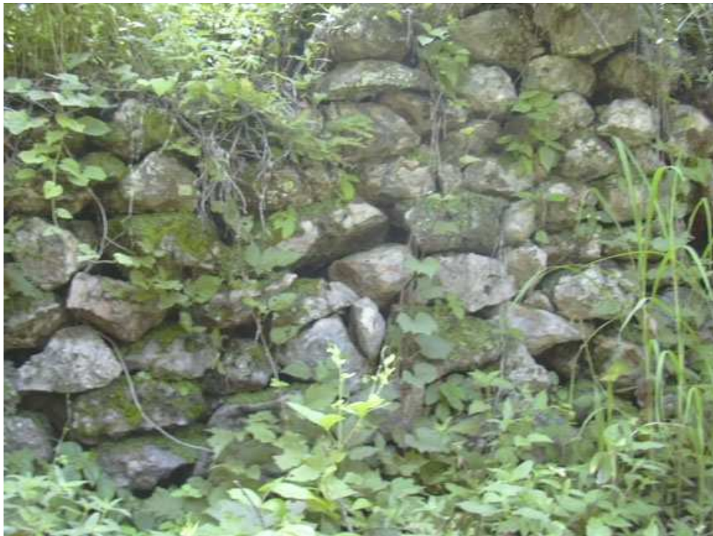
Figure 9. Yichkuhuan, Terrace wall.
