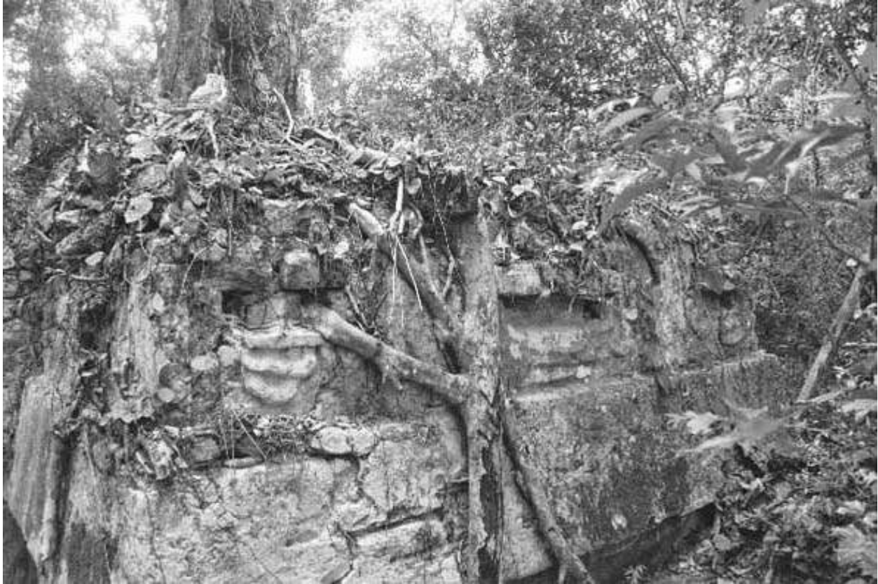
Figure 13. Detail of the frieze and removed vegetation on Building B, Group II.
