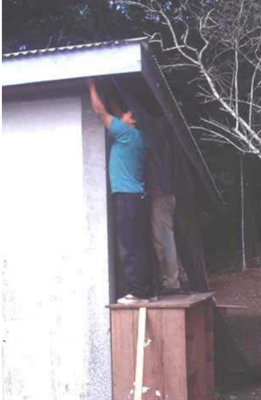
Figure A1:12. Federico and Israel installing screening.
