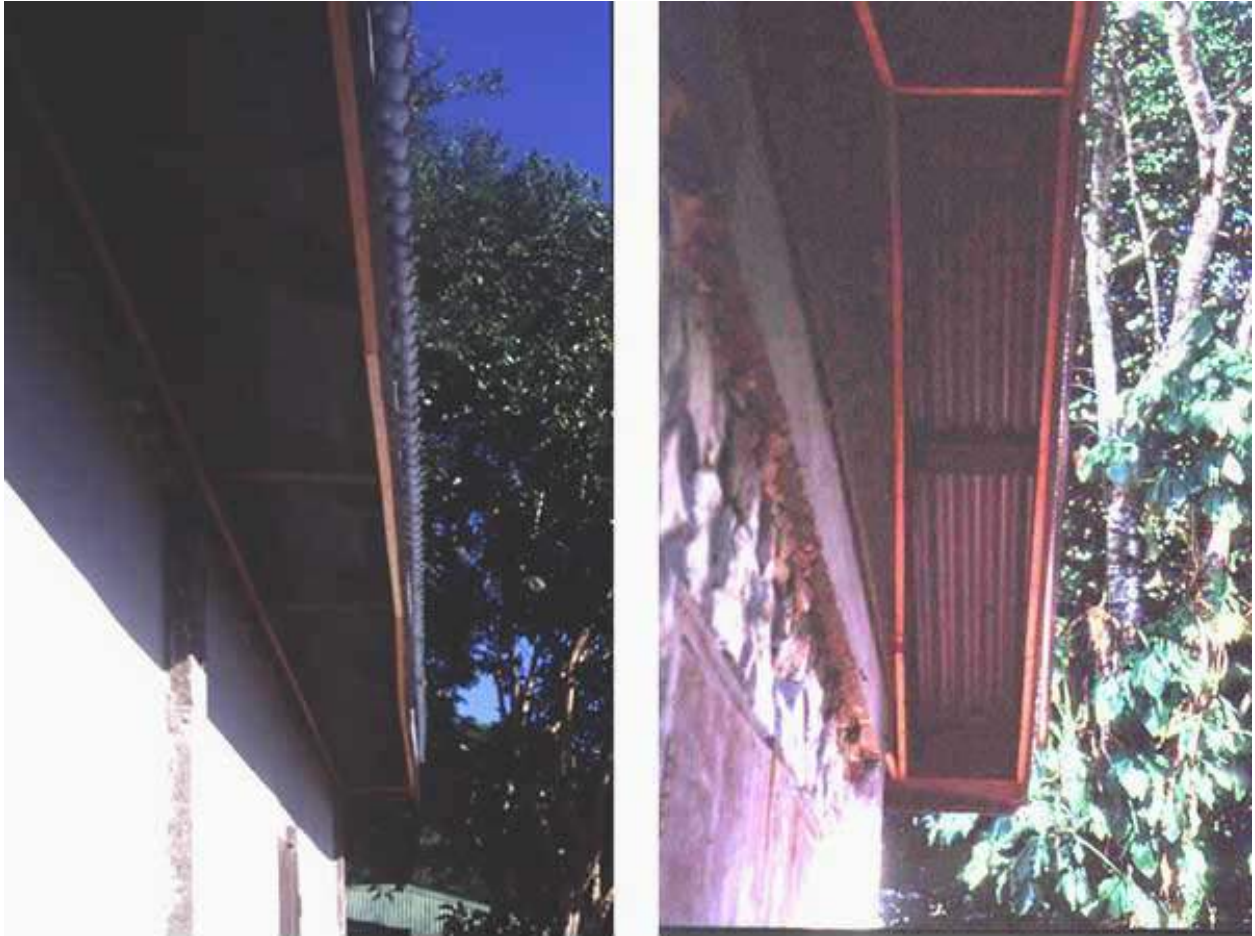
Figure A1:11. Bodega soffit after screening.
