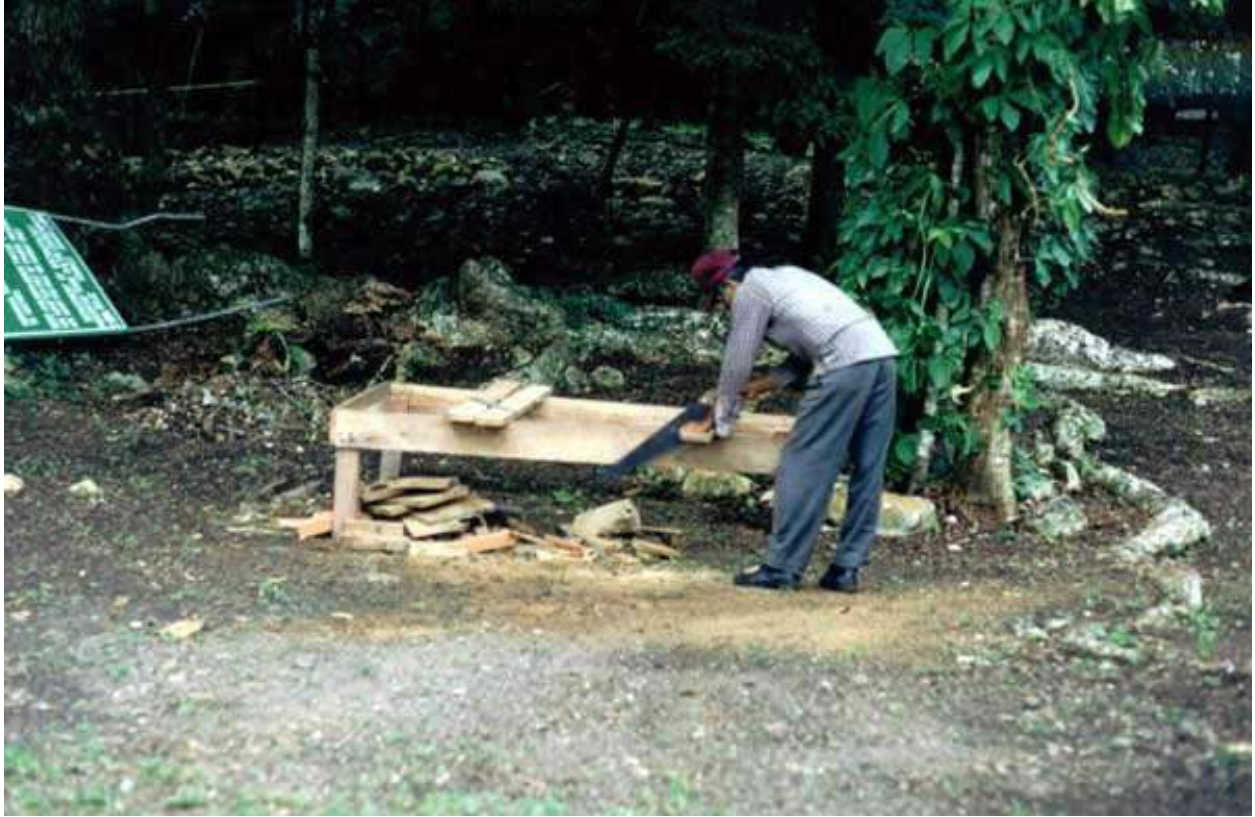
Figure A1:8. Israel at work on the new shelving.
