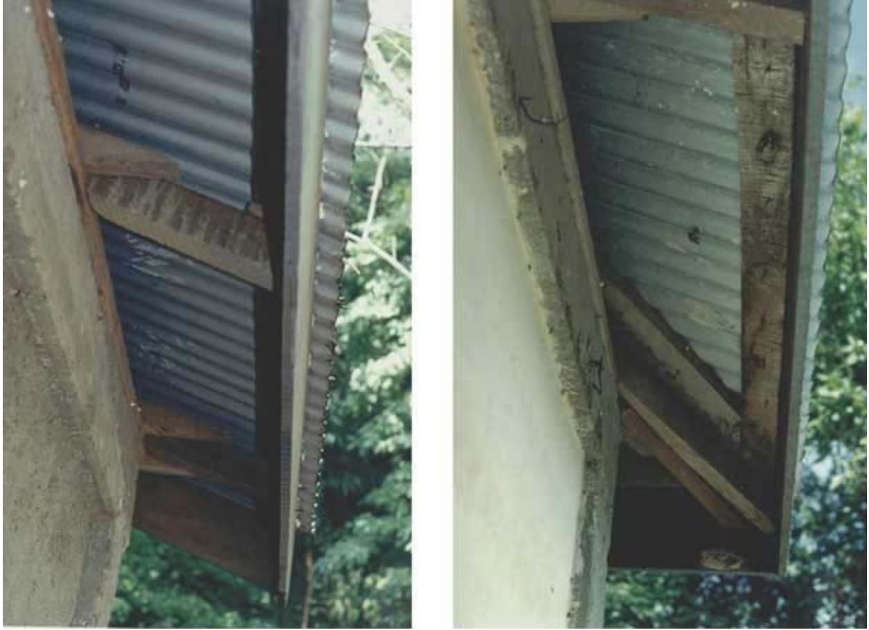
Figure A1:10. Bodega soffit before screening.
