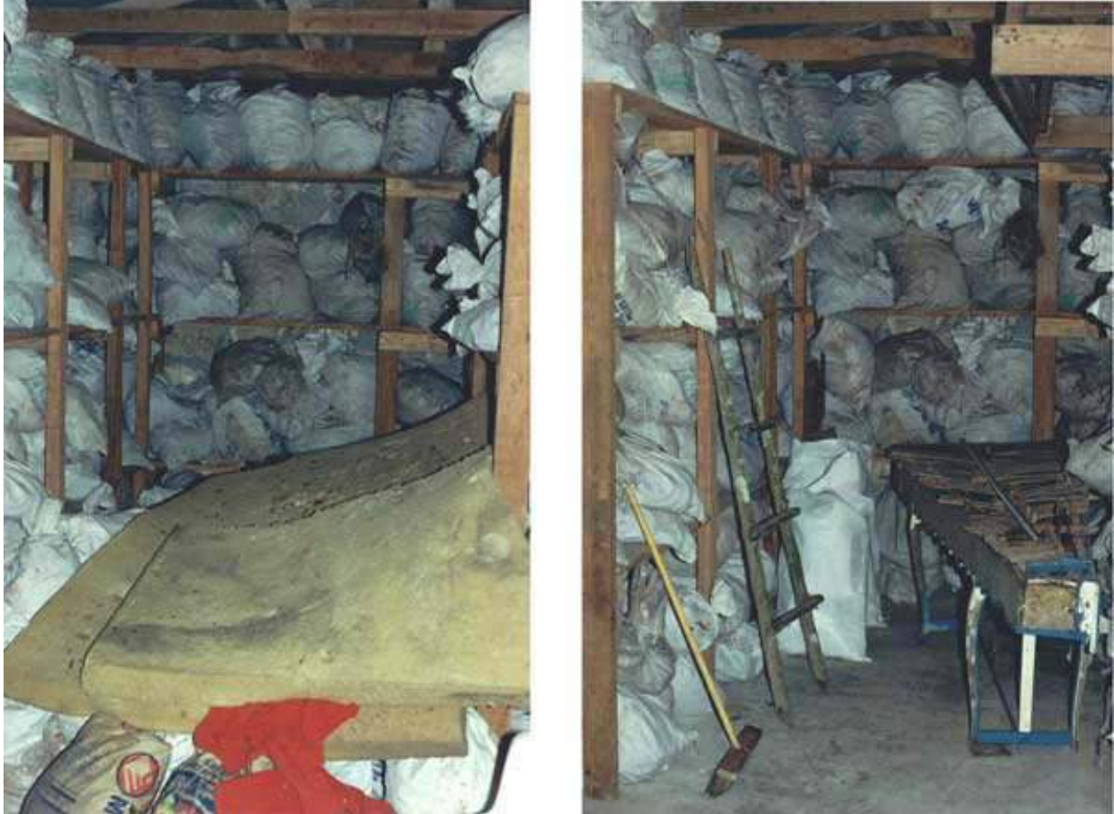
Figure A1:2. Shelving to the left of the bodega door, before (left) and after (right).
