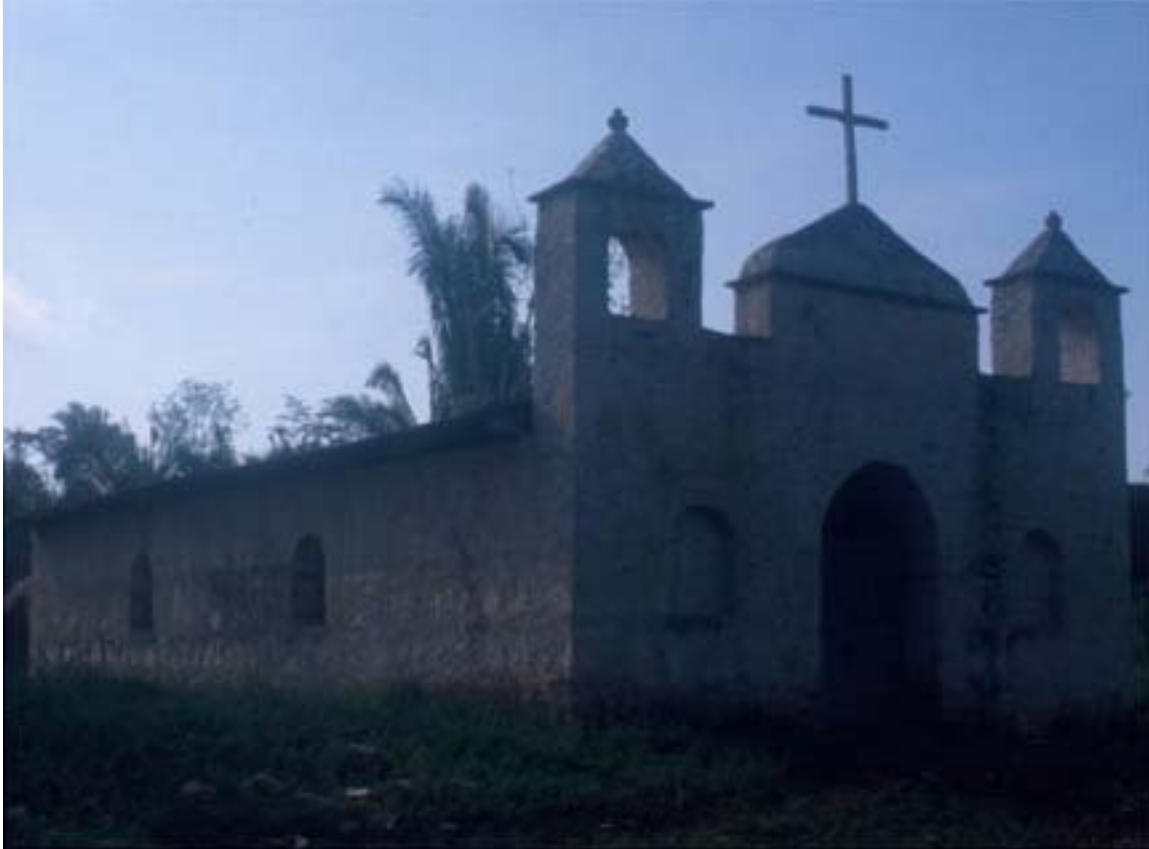
Figure 11. The recently completed church in modern La Caoba, built in part from fill material taken from remains of ancient Maya structures.
